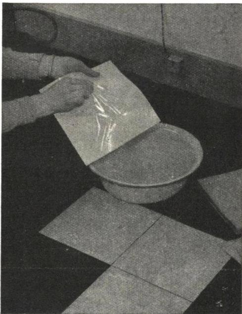
parent film protecting the adhesive; the tiles must be immersed in water for about 30 seconds, and then the protective film can be readily removed. Pressure on the face of the tile, when in position, brings about an almost immediate fixing.
